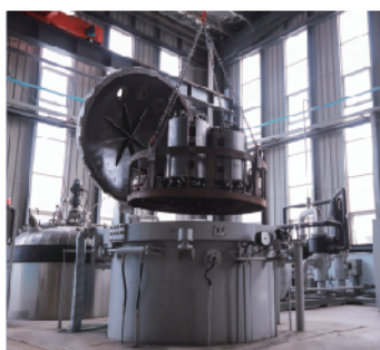
VACUUM PRESSURE IMPREGNATION
